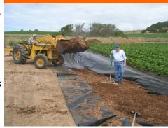
The bioreactor treats agricultural runoff through the action of denitrifying microbes that convert nitrate to nitrogen gas. Microbes live on the woodchip and pond liner surfaces and their growth is stimulated by the carbon contained in the woodchips. The woodchips are anticipated to last for 10-15 years, before requiring replacement.
